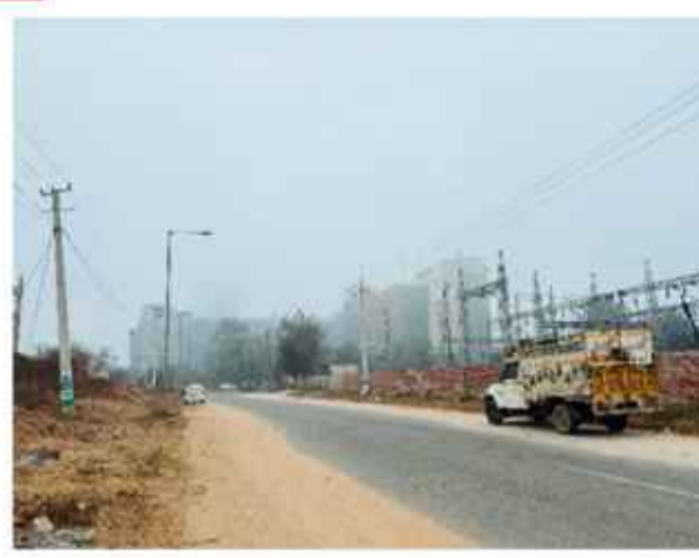
View at 1, power station and access road
